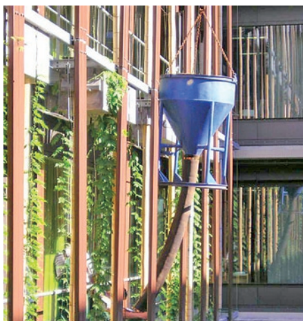
The filling of plant troughs
