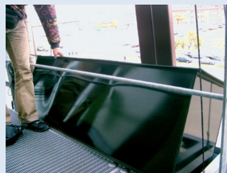
An example of planter insulation at the Physics building in Adlershof: exterior: fibre-cement concrete; several centimetres of insulation and a plastic inner planter for the planting
