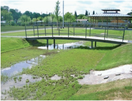
Rainwater management at the new building of the Technical Vocational College (Oberstufenzentrum Bautechnik II/Holztechnikconstruction) in Pankow, Berlin
