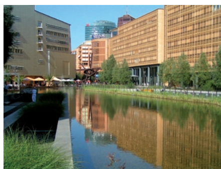
Roof greening, rainwater usage und urban bodies of water at Potsdamer Platz Berlin (Priorities 2, 6 and 3 in combination)
