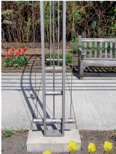
Left: An example of a durable, stable climbing support made of stainless steel
