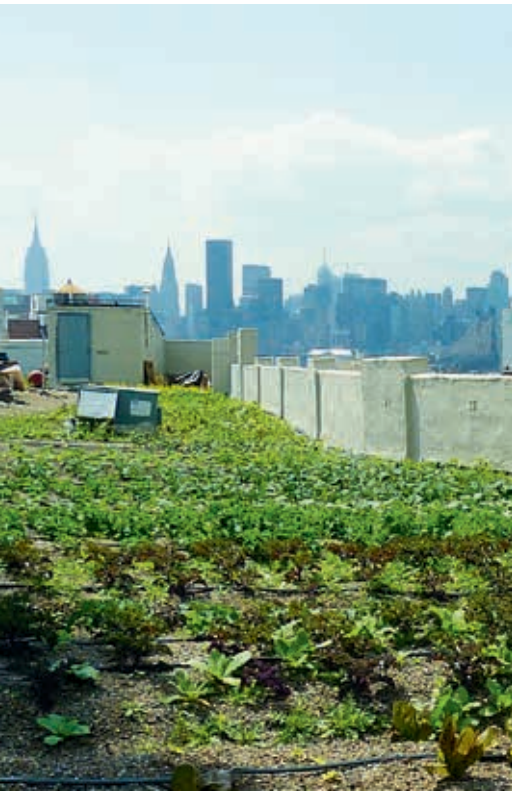
Brooklyn Grange is a 4,000 m 2 rooftop farm on a former factory building in New York City, USA.
