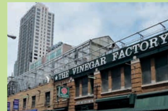
The New York delicatessen supplier Eli Zabar grows tomatoes, lettuce and bell pepper in greenhouses on the roof of a supermarket. The products are sold and processed in the adjacent supermarket and restaurant. The waste heat from the bakery is used to heat the greenhouse.
