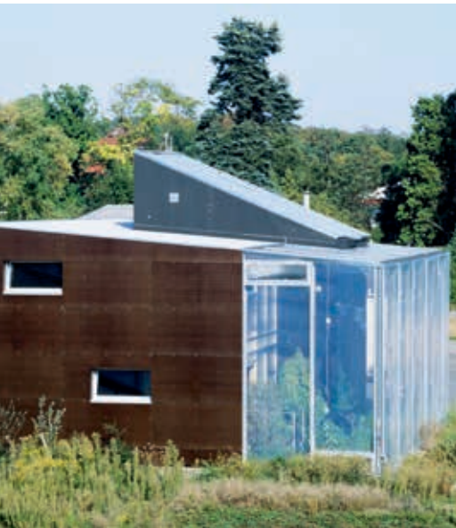
Watergy building prototype in Berlin with a greenhouse as a humid air solar collector. Here, the greenhouse acts as heating for the building. Warm, humid air from the collector is dried and either fed straight into the building's heating system or stored for later use.
